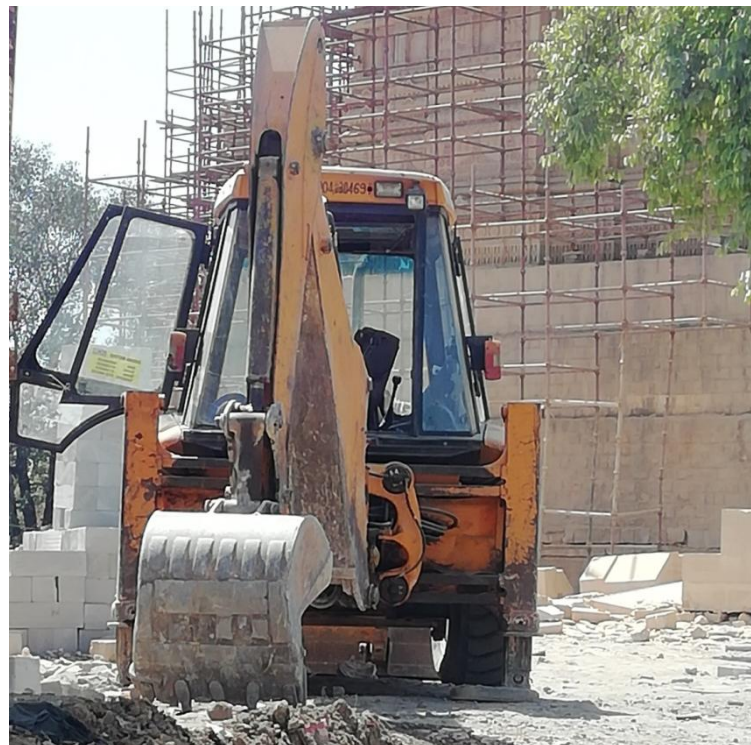
Figure 1: JCB Machine Equipment at Construction Site
