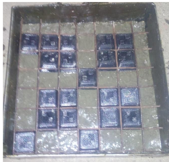
Casting of U-boot Block
