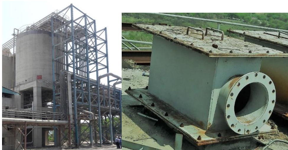
Fig. 3a Silo mounting, Target box Vent box with bag filters arrangement.
